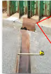
Main Street over B&A Railroad Beckett, MA
